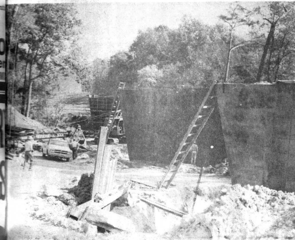
NOVEMBER 3 — The third support of the massive bridge under construction south of Sadsad Ridge in Tishomingo County is nearing completion. The foundations of the bridge are being laid. The bridge construction is a portion of the work under way on the Natchez Trace parkway which runs through Tishomingo county. It is under tentative discussion as to which section of the Trace will be started in the future in the northern counties of the state.
